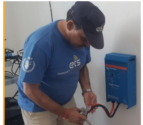
ETS staff installs solar power equipment in the Security Operations Centre (SOC) in Dikwa. Photo: WFP/ETS
