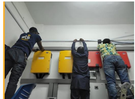
The ETS installed a back-up solar power system at the Red Roof hub in Maiduguri. Photo: WFP/ETS
