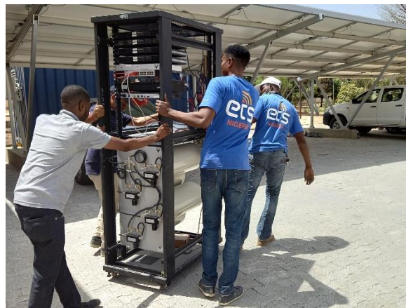
ETS relocate security telecommunications equipment in Maiduguri.
