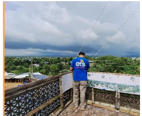
The ETS installs data connectivity at Kutupalong Registered Camp 2. Photo: WFP/ETS
