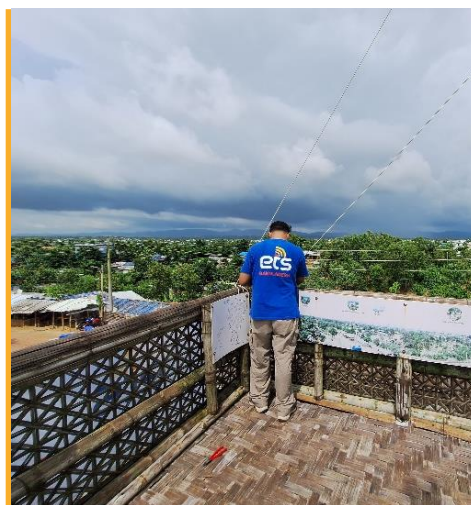
The ETS installs data connectivity at Kutupalong Registered Camp 2. Photo: WFP/ETS
