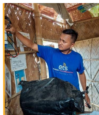
The ETS installs a router at an IOM Shelter Management and Shelter Development site in Camp 12. Photo: WFP/ETS
