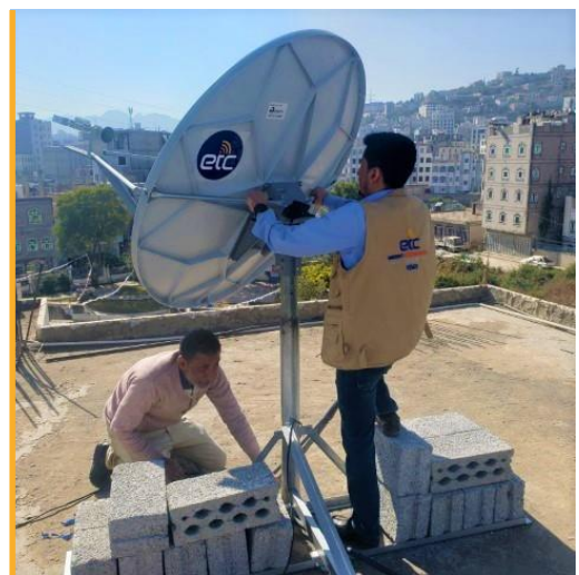
The ETC is installing a dedicated VSAT station for the INGOs hosted by Save the Children International (SCI) in Ibb to provide stable and secure connectivity. Photo: WFP/ETC
