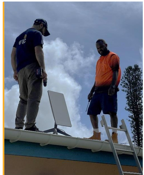
The ETC installs a Starlink satellite data device at Tafea PEOC, Tanna Island, for use in communication between PEOC and the NDMO HQ in disaster response. Photo: WFP/ETC
