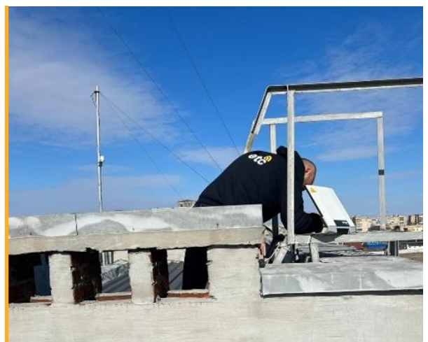
The ETC continues to optimize installed Starlink VSAT terminals in Ukraine for greater performance. Photo: WFP
