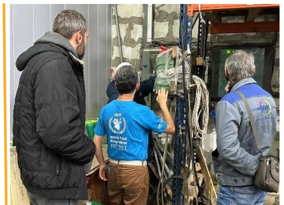
The ETC supports installation of a fibre optic cable to provide connectivity to UN responders in the Logistics Cluster warehouse in Dnipro. Photo: WFP/Hafeez Esaqzai
