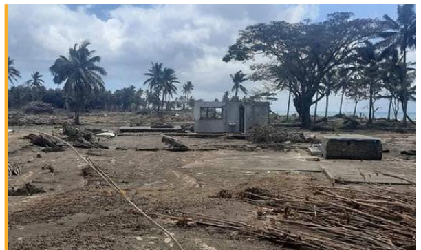
Damage caused in Tonga's capital, Nuku'alofa, by the volcano eruption and subsequent tsunami on 15 January 2022. Photo: © UNICEF/Consulate of the Kingdom of Tonga.
