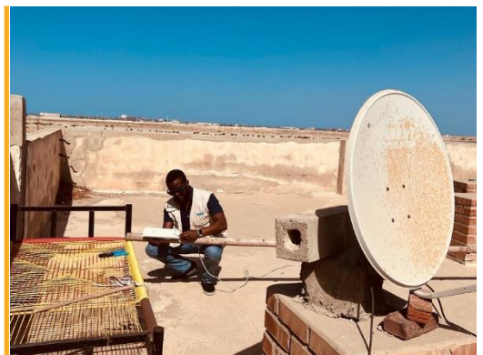
A WFP IT specialist connects the shared I/NGO office hosted by Welthungerhilfe to the ETC satellite connectivity network in Port Sudan.
