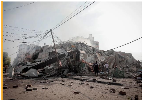
Telecommunications and power infrastructure have been destroyed in Gaza due to the ongoing conflict. Photo: Getty Images/Momen Faiz.
