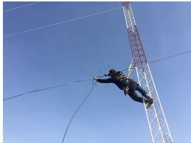
Habib Shashati, ETC's security telecommunications specialist, installs a radio repeater in As Salamiyah. Photo: WFP/ Erika Iglesias
