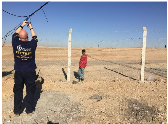
The ETC finalises the deployment of security telecommunications services in As Salamiyah. Photo: WFP/ Erika Iglesias
