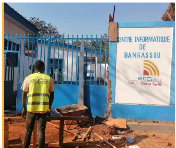
Construction work on the ETC Learning Centre and Cyber Café in Bangassou is finalised before the launch of the service. Photo: WFP/ ETC
