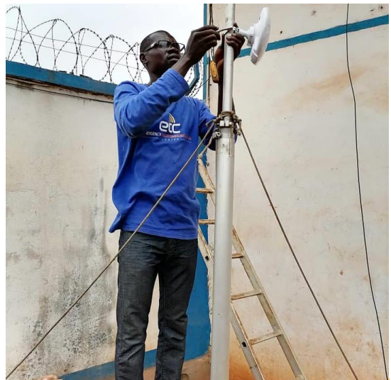
An ETC technician adjusts equipment for improved connectivity in Batangafo,
