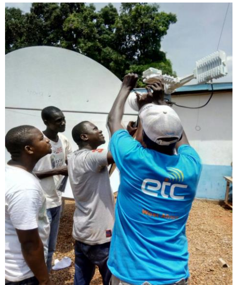
Sam Okudi, ETC telecommunications specialist installs a satellite kit at the IMC office to provide shared internet connectivity to humanitarian in Bria. Photo credit : ETC CAR.
