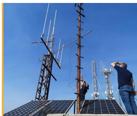
The UHF radio repeater in Hatay is now restored for security communications services. Photo: WFP/ETS
