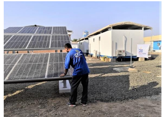
A member of the ETC team checks a solar panel installed at the UN hub in Al Mokha. Photo: WFP/ETC
