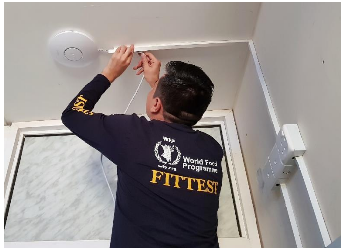
Abdullah Ayoubi from FITTEST supporting the deployment of the EOC in Aden. Photo: ETC Yemen
