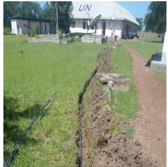
ICT staff setting cable underground for Bor sub-office, South Sudan.
