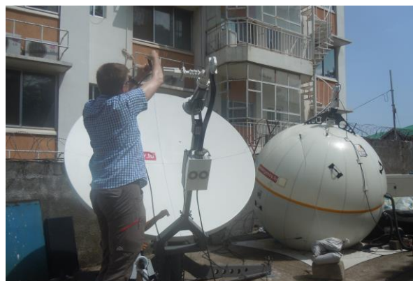
ETC partner, Ericsson Response, installing a satellite kit at WFP Country Office in Sierra Leone.
