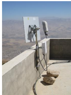
ETC radio repeater in Sulaymaniya, Iraq. Source: Khawar Ilyas, WFP.
