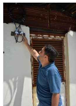
Assessing telecoms and IT connectivity at the UN hub in Gaziantep, Turkey. Source: Salma Farouque, WFP.
