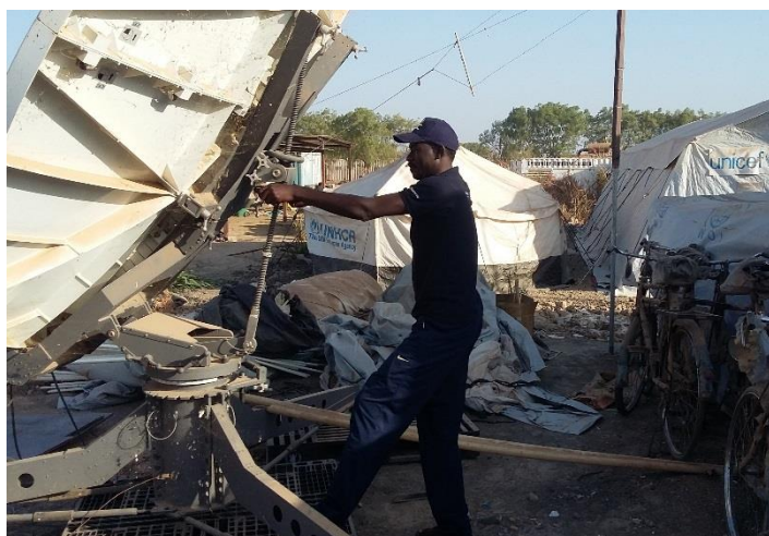
ETC Technician John Mawa performing VSAT connectivity infrastructure changes in Bentiu (Unity State)
