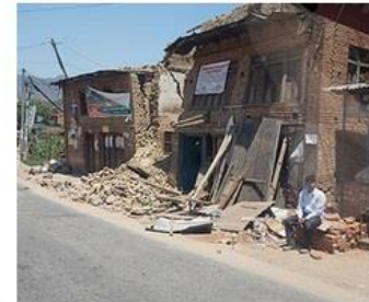
Destruction caused by the April 25 earthquake. Photo: WFP/ Rob Buurveld
