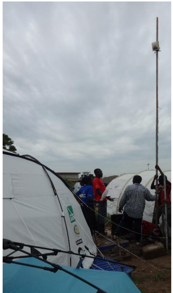
Installing the wireless transmitter in UNHCR compound, in Yida, Unity State.
