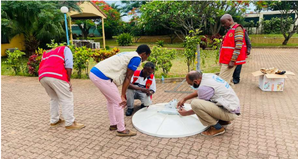
ETC–WFP country team setting up a satellite dish. Photo Credit: Emergency Telecommunications Cluster
